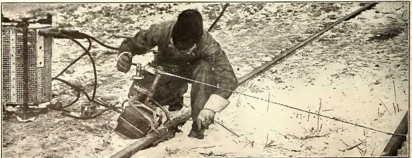
PORTABLE ELECTRIC WELDER IN USE UNMOUNTED
